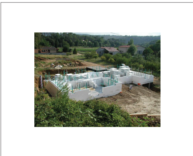
Figure 4 Construction site with trestles
